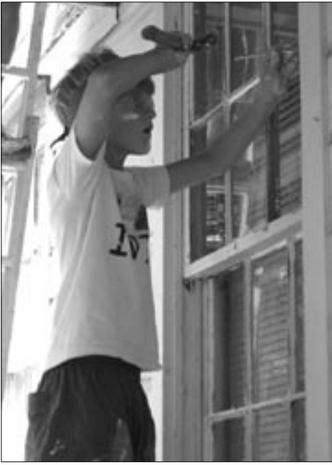
The youth of Grace Church, Charleston attended a Homeworks Session in Columbia, South Carolina in June. Above is Grace's John Black repairing windows. The group was joined by fifty youth from across South Carolina and Columbus, Georgia. They repaired homes and cleaned up yards.
