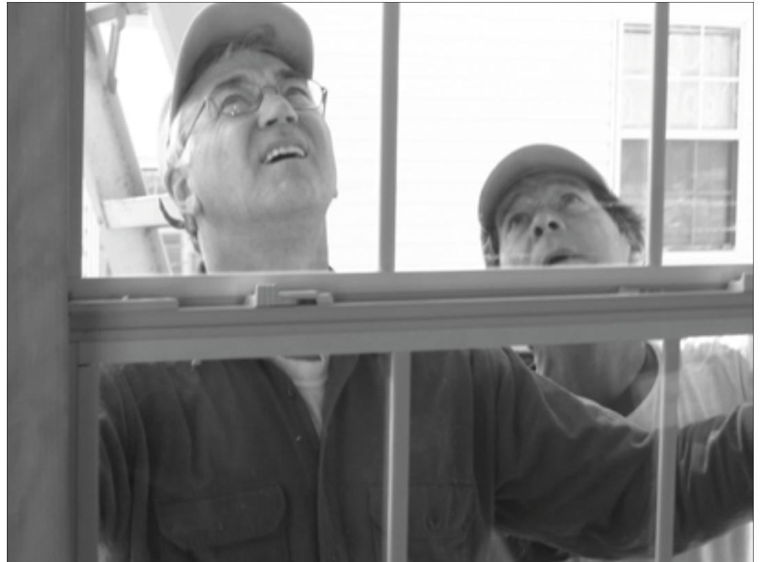
Jim Berry and Jim McClary, pictured above, work on seating and squaring a window.
